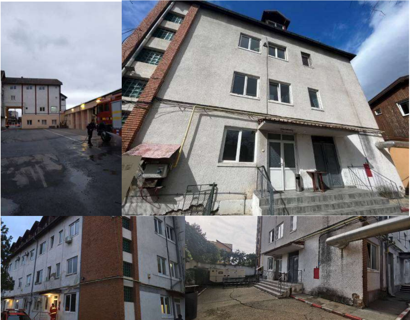
Figura 7 C1 Administrative building of SESI and SFD
